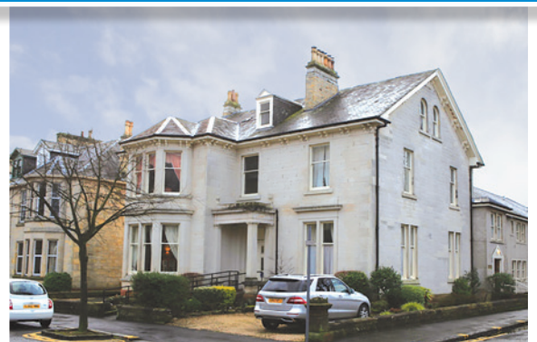
HOWARD HOUSE, KILMARNOCK
